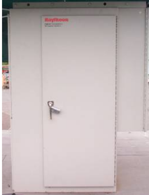
Figure 3.4.6-2 Integrated Roadside Unit. This small cabinet provides an environmentally-conditioned home for all tolling point cable termination, processing and communications equipment.
