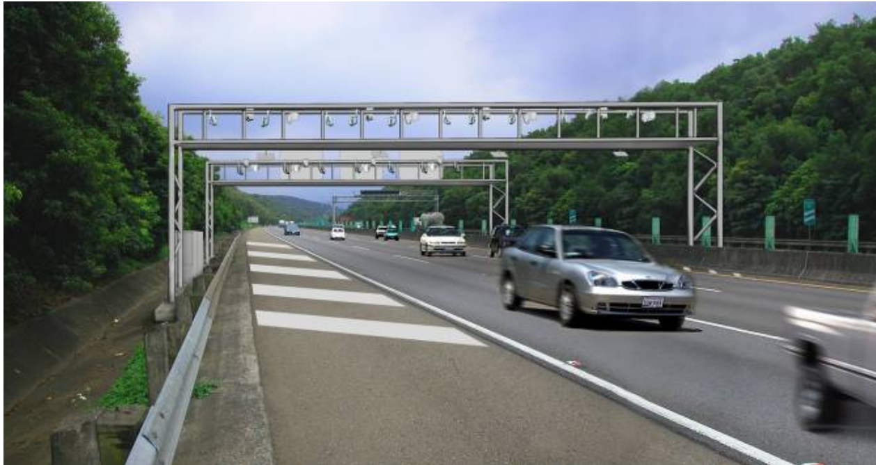
Figure 3.4.8-1 Standard Gantry. The standard Truss structure simply and adequately supports tolling zone equipment.
