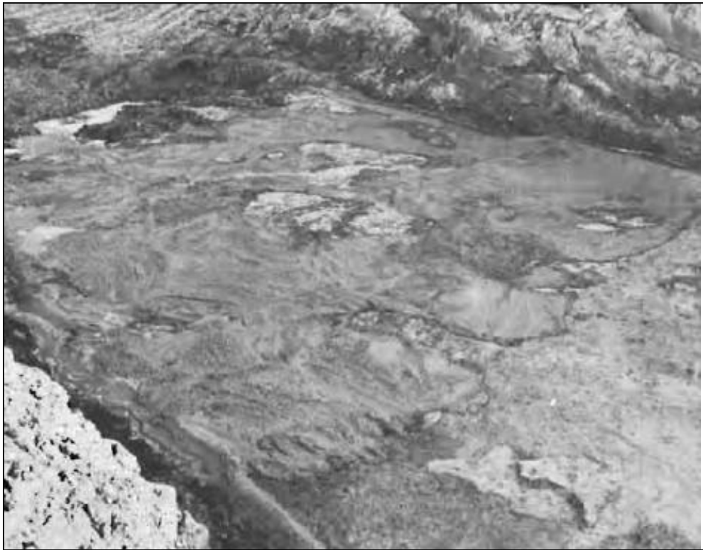
Figure I-4-5. Rock Foundation in Cutoff Trench after Dental Concrete Treatment
