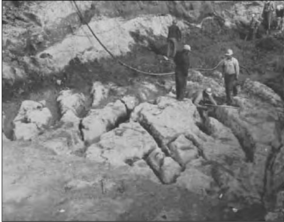
Figure I-4-4. Typical Limestone Foundation Joints
